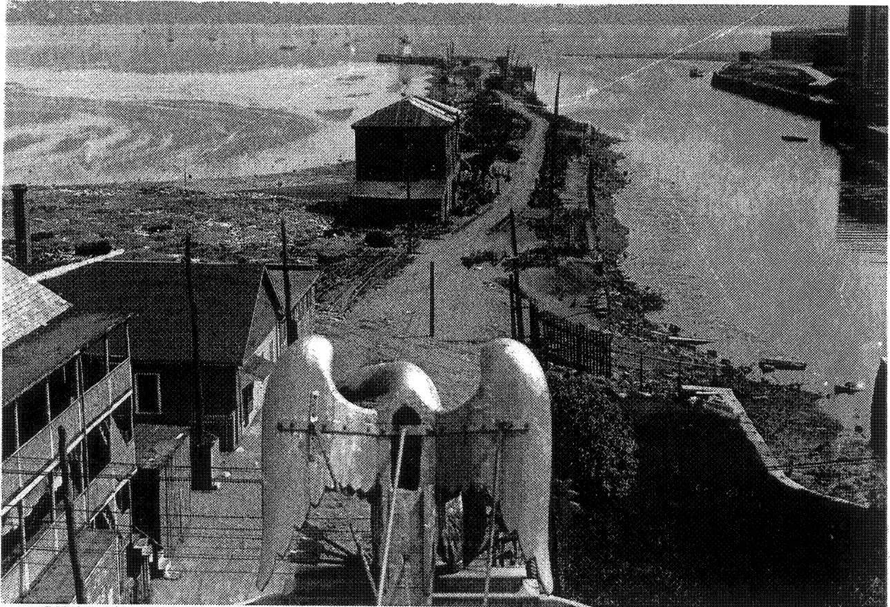
Figure VI.2. View of Derby Wharf Looking South from the Top of the Custom House, ca. 1930 (Peabody Essex Museum Collection, neg. 9616).
